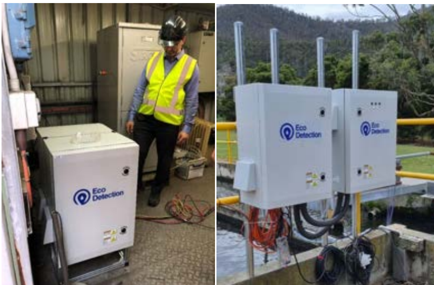
Figure 1b: Installation examples of Eco Detection units. Left: Norske Skog, device on frame, access to mains power. Right: Sewage treatment plant outfall, TasWater, Turriff Lodge (New Norfolk), device mounted to railing with access to mains power.
